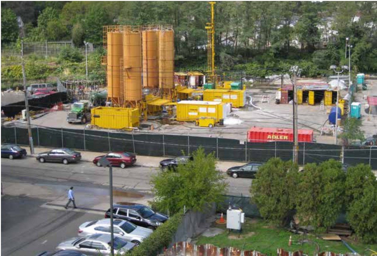
Fig. 10. PACCHIOSI Jet Grouting plant installations.
