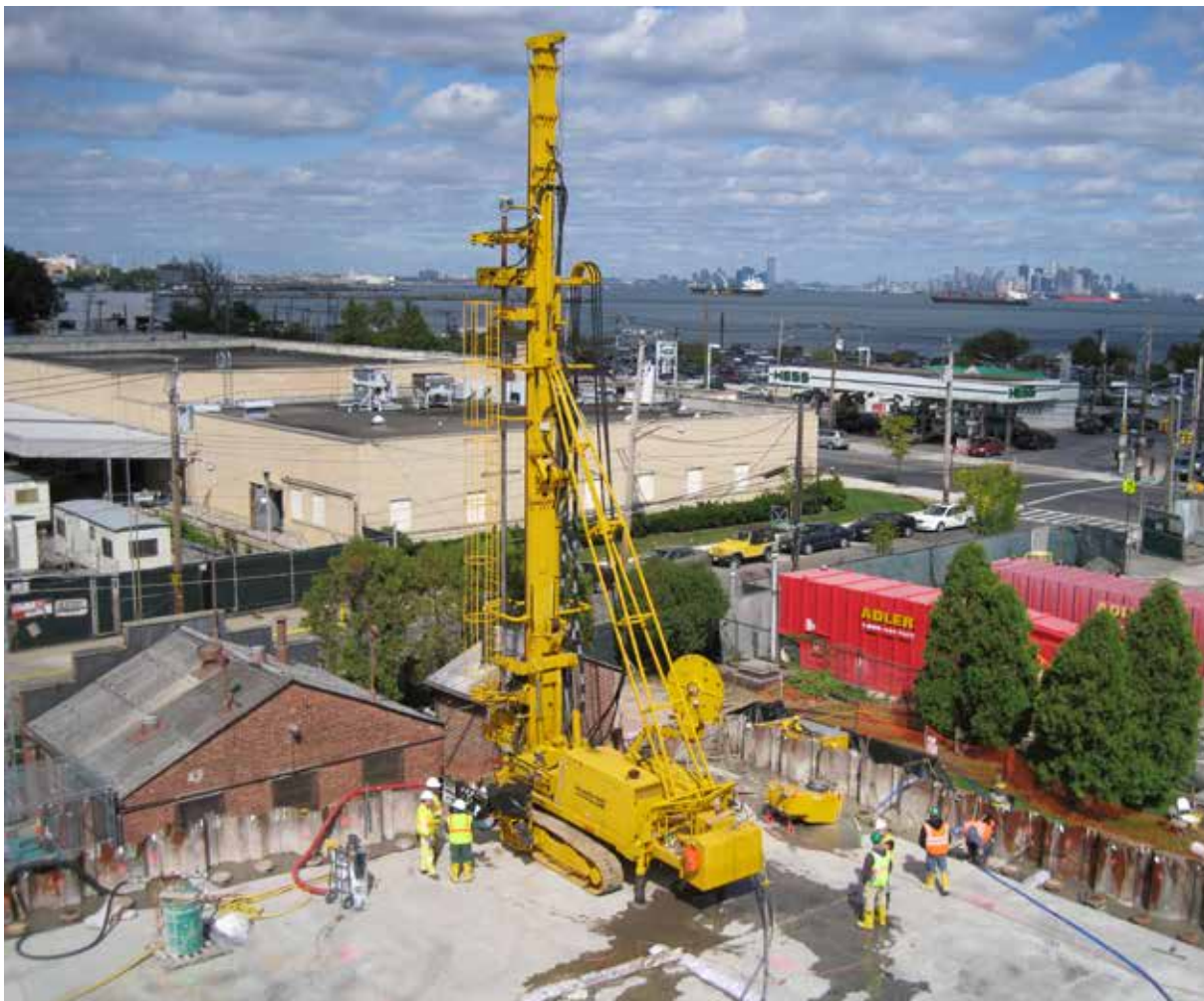
Fig. 1. Former Clifton OU-1 MGP site.
