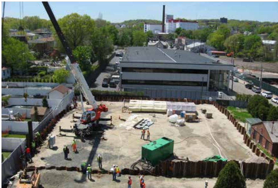
Fig. 2. Perimetral shallow steel sheetpiling .
