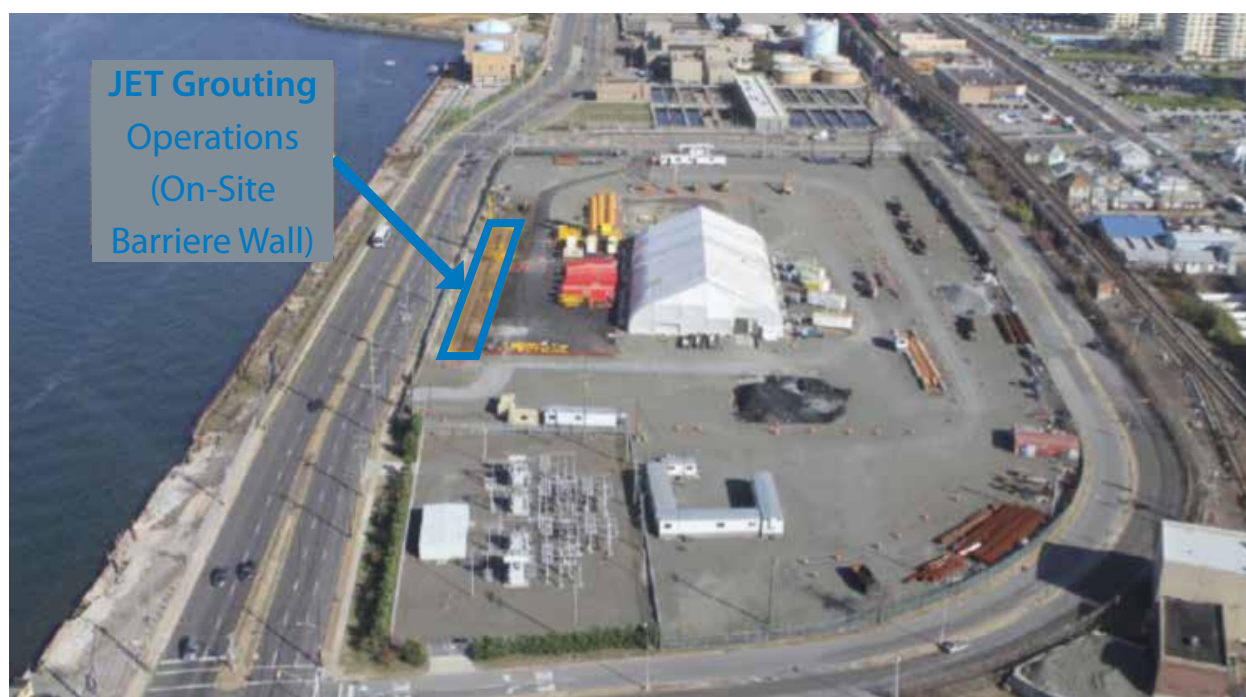
Fig. 3. View of Rockaway Park MGP area during works
