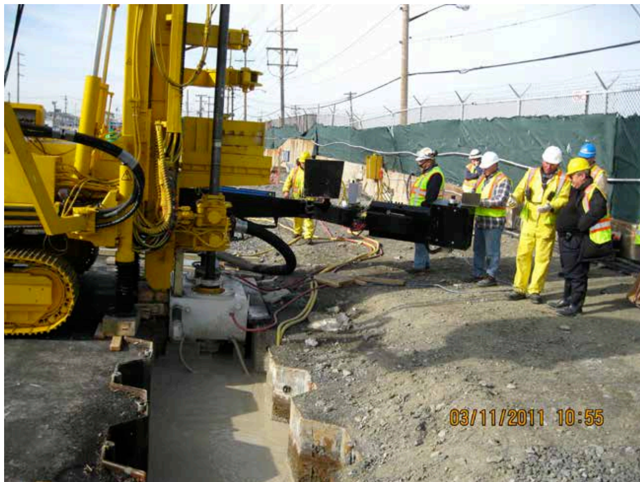
Fig. 6. Special watertight tank used for Jet Grouting spoils' collection
