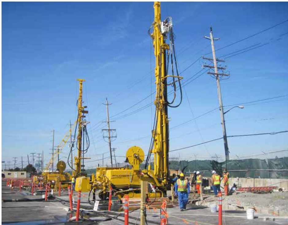
Fig. 5. PACCHIOSI P1500ECS drill rigs operating with automatic rod loader
