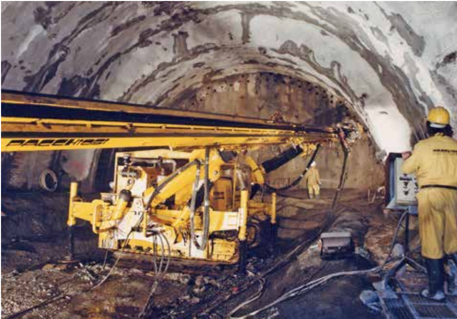
Fig. 4. P1500 TAF hydraulic drill rig employed for dome consolidation.
