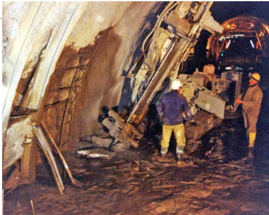
Fig. 9. PRP 105 drilling machine during consolidation of piers and micropiles.
