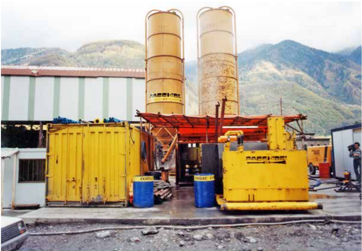
Fig. 10. Mixing and injection installations.
