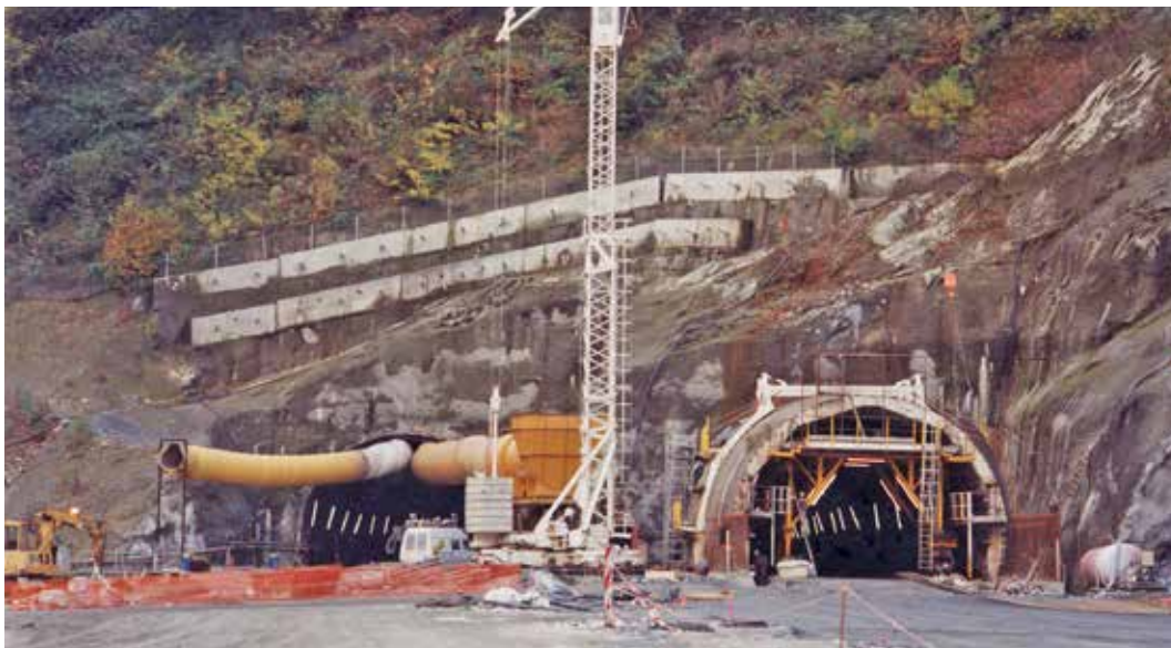
Fig. 2. Entrance of Des Hurtieres tunnel, eastbound and westbound tubes.
