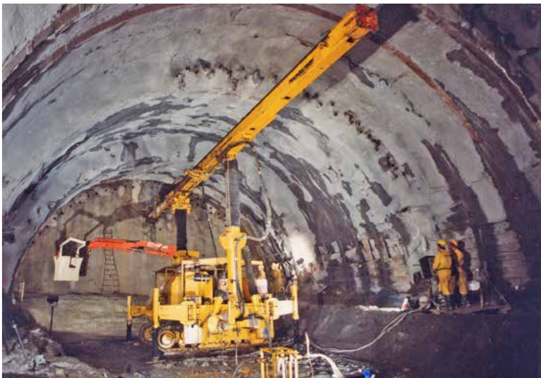
Fig. 7. P1500 TAF drilling machine during consolidation of the excavation front.
