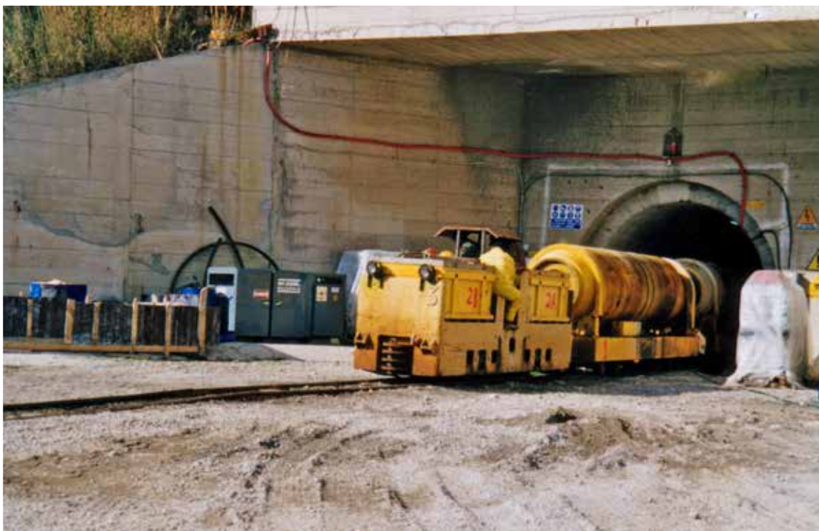
Fig. 5. Movement of the concrete in the tunnel for pouring.
