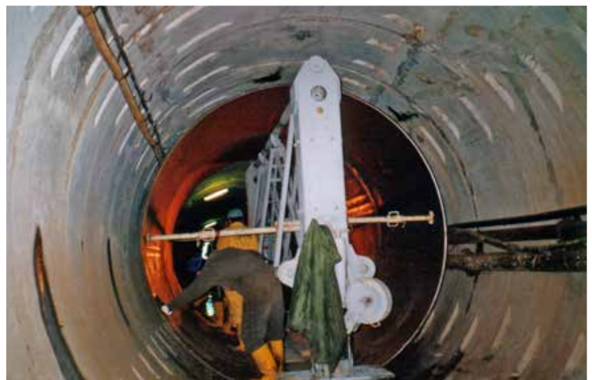
Fig. 9. Installation of pipe in the tunnel and injection.
