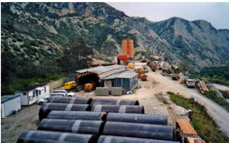
Fig. 10. View of the worksite.
