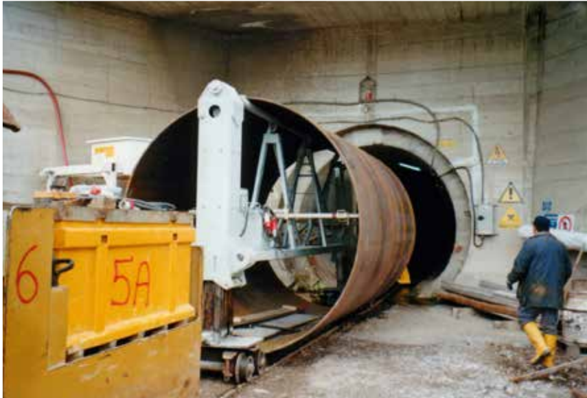
Fig. 8. Movement of the pipe into the tunnel.
