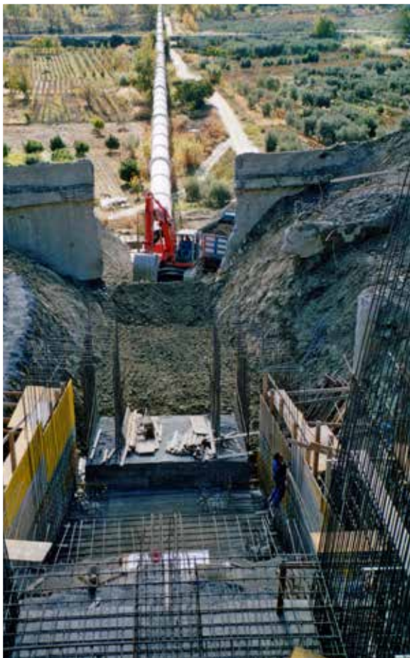
Fig. 11. Construction of the tank.
