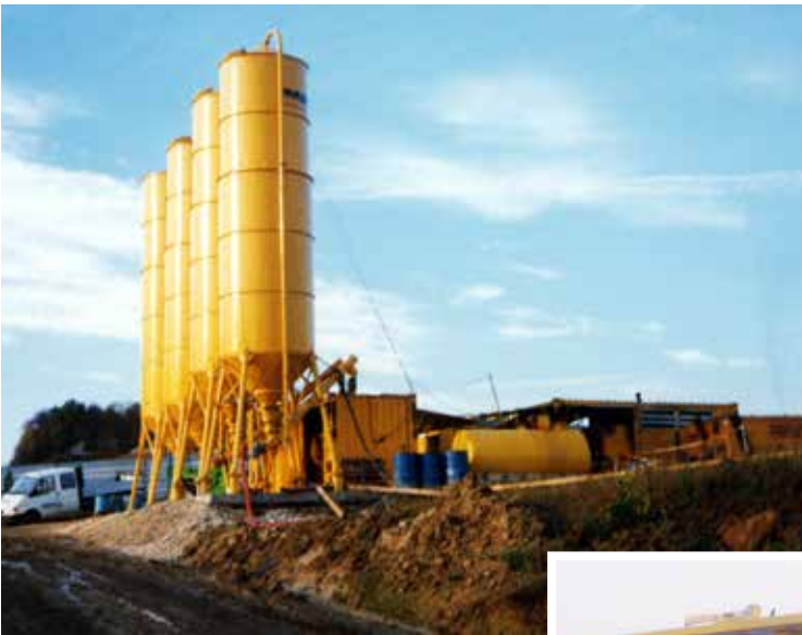
Fig. 8. View of the worksite.
