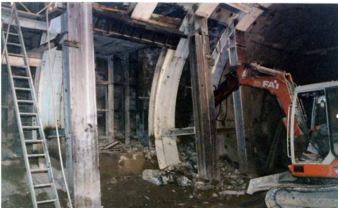
Fig. 10. Intertube: stage of controlled demolition of final covering slabs.
