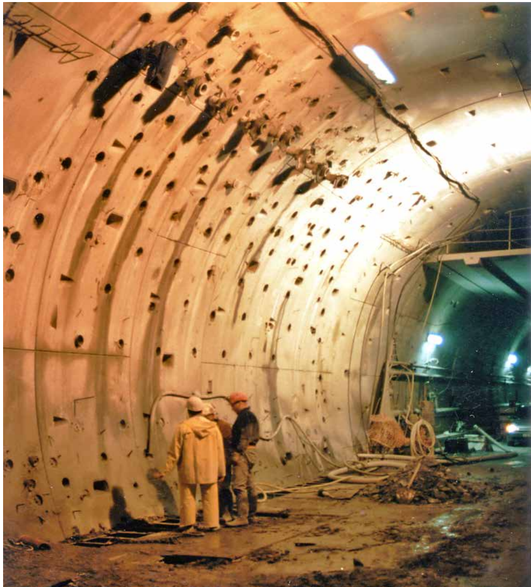
Fig. 9. View of the wall prepared with preliminary holes and preventers.
