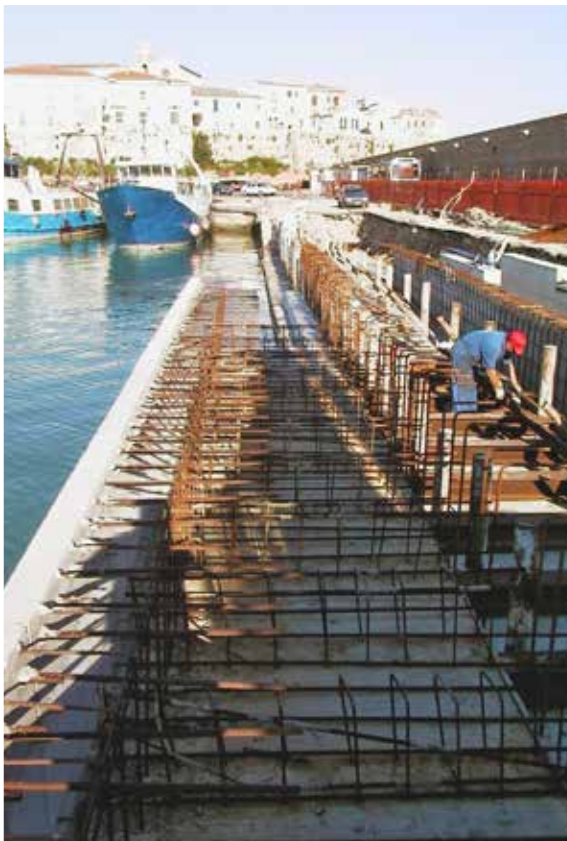
Fig. 8. Detail of the micropile heads
