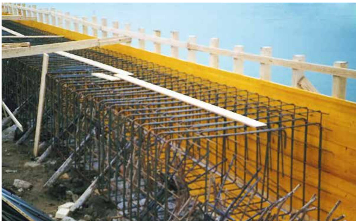
Fig. 14. Reinforcement and carpentry of the bar.
