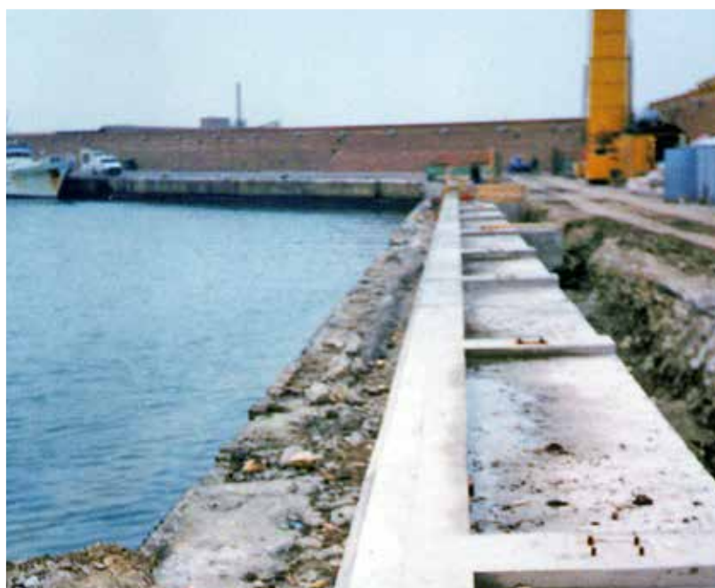
Fig. 14. Reinforcement and carpentry of the bar.
