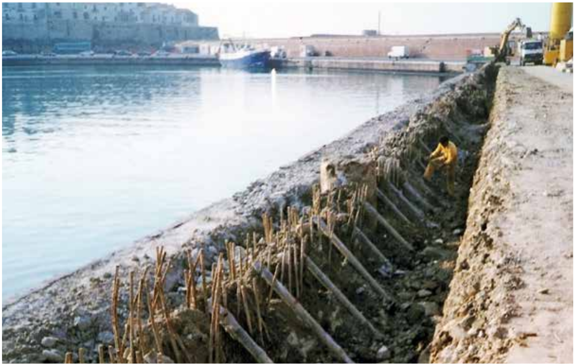
Fig. 13. Detail of the pile and micropile heads
