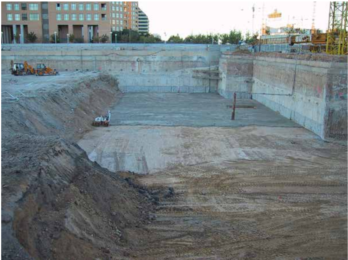
Fig. 11. Excavation of the foundation.
