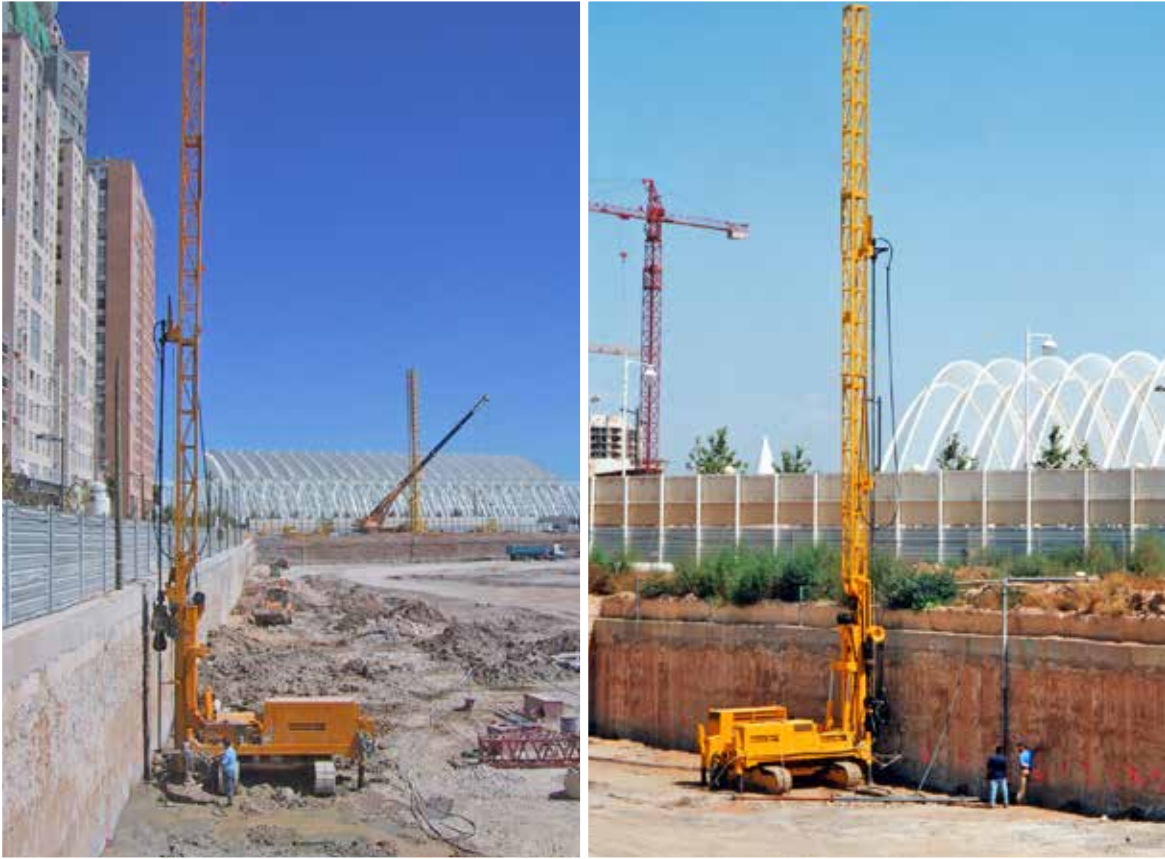
Fig. 9 - 10. P 1500 EC drill rig performing Jet Grouting.
