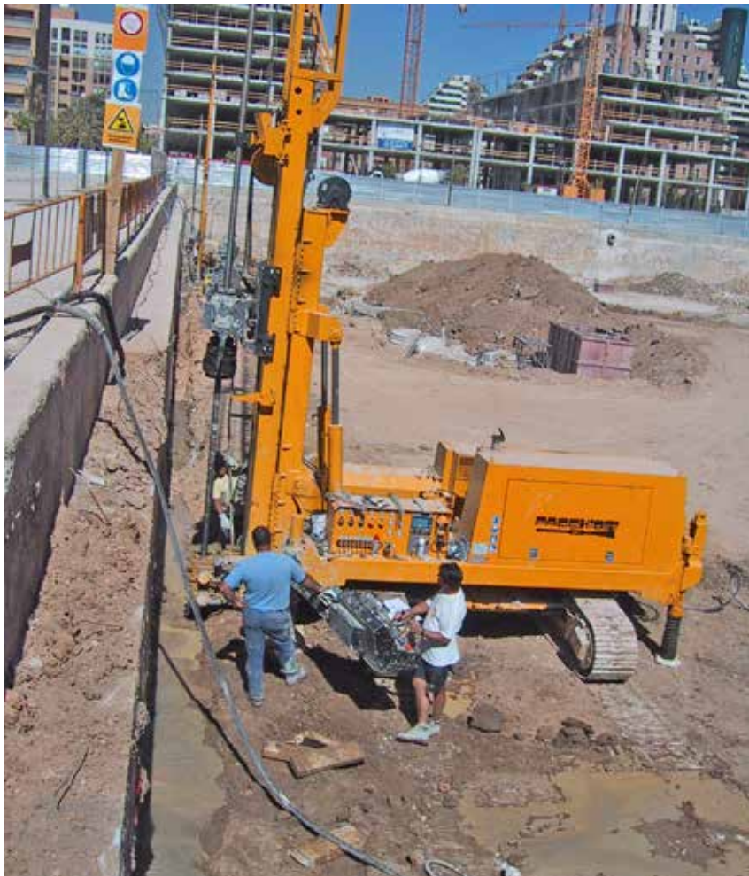
Fig. 9 - 10. P 1500 EC drill rig performing Jet Grouting.
