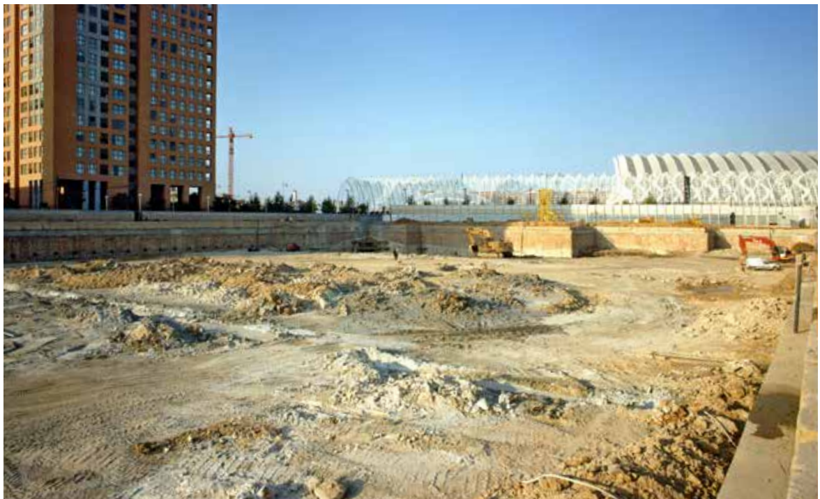
Fig. 3. Fondazione area of the new courthouse.
