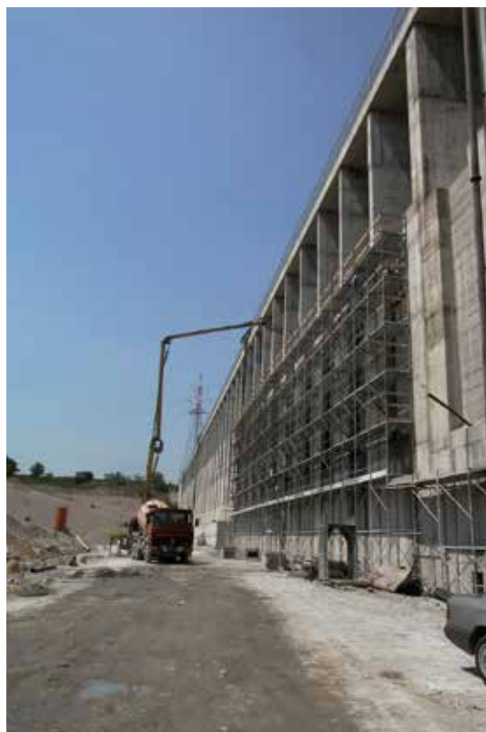
Fig. 3. Pouring of concrete between the panels.
