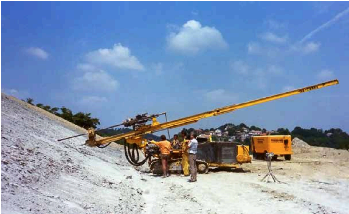
Fig. 5. Insertion of Cloujet nails after excavation.
