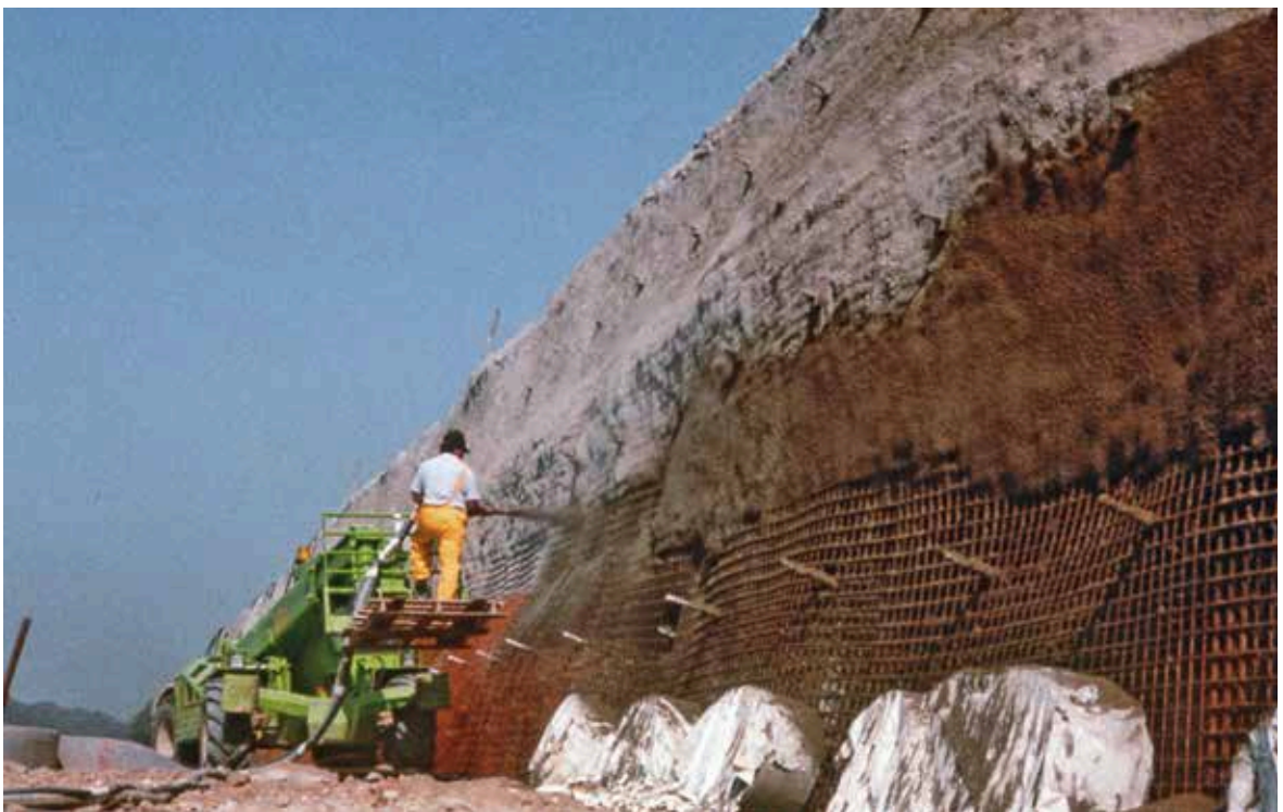
Fig. 7. Pouring of the enclosing walls after installing the reinforcement.
