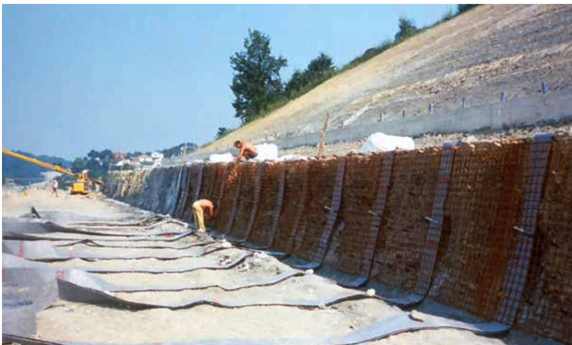
Fig. 6. Installation of electrically welded screen.
