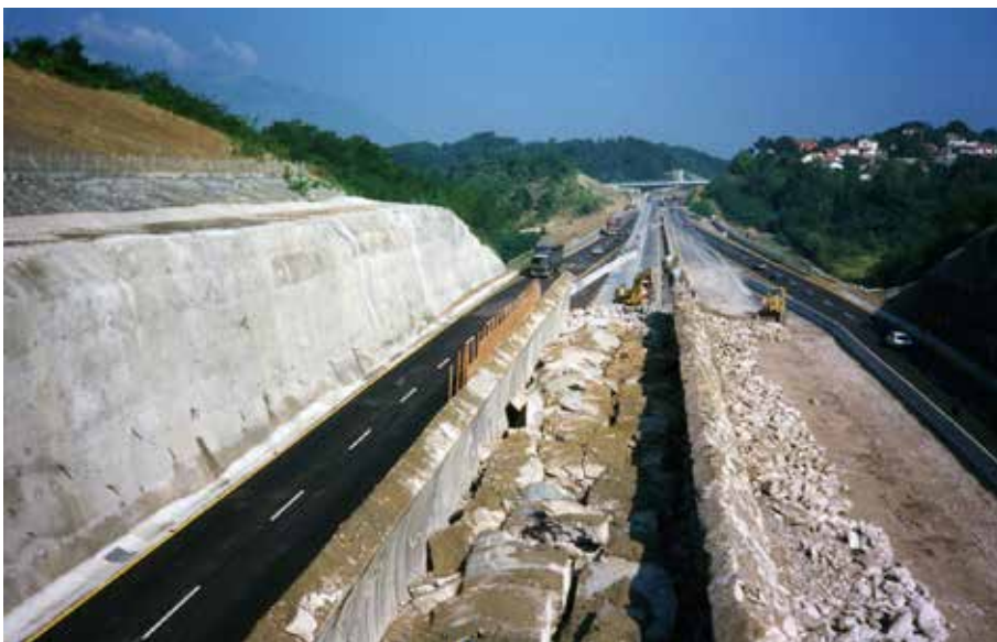
Fig. 10. Demolition of the tunnels.
