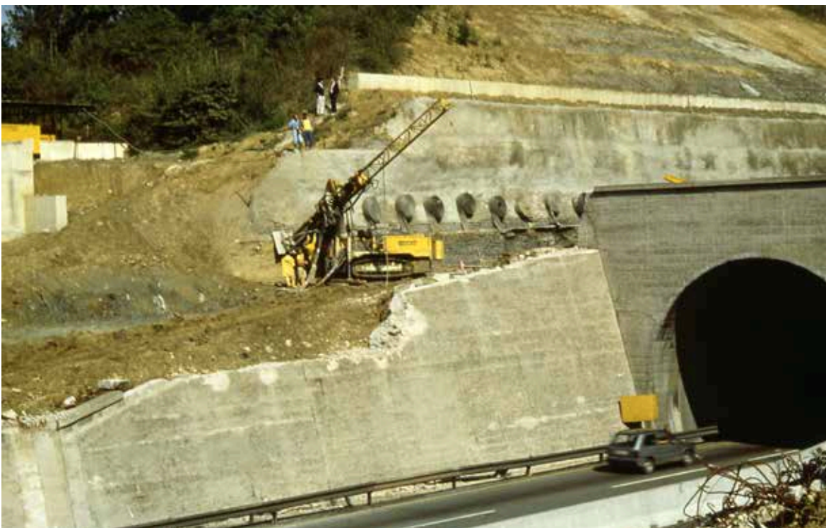
Fig. 8. Subsequent stage of insertion of cloujet nails.
