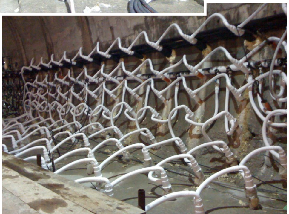
Fig. 13. Overview of the fields at the start of freezing
