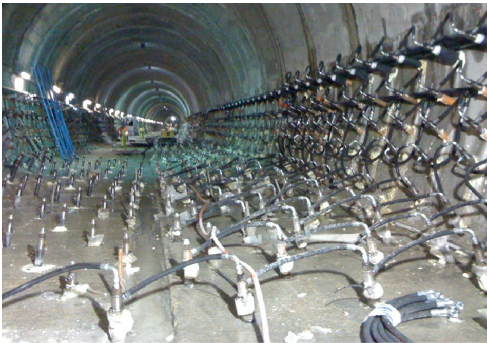
Fig. 12. Overview of the fields equipped but not frozen.
