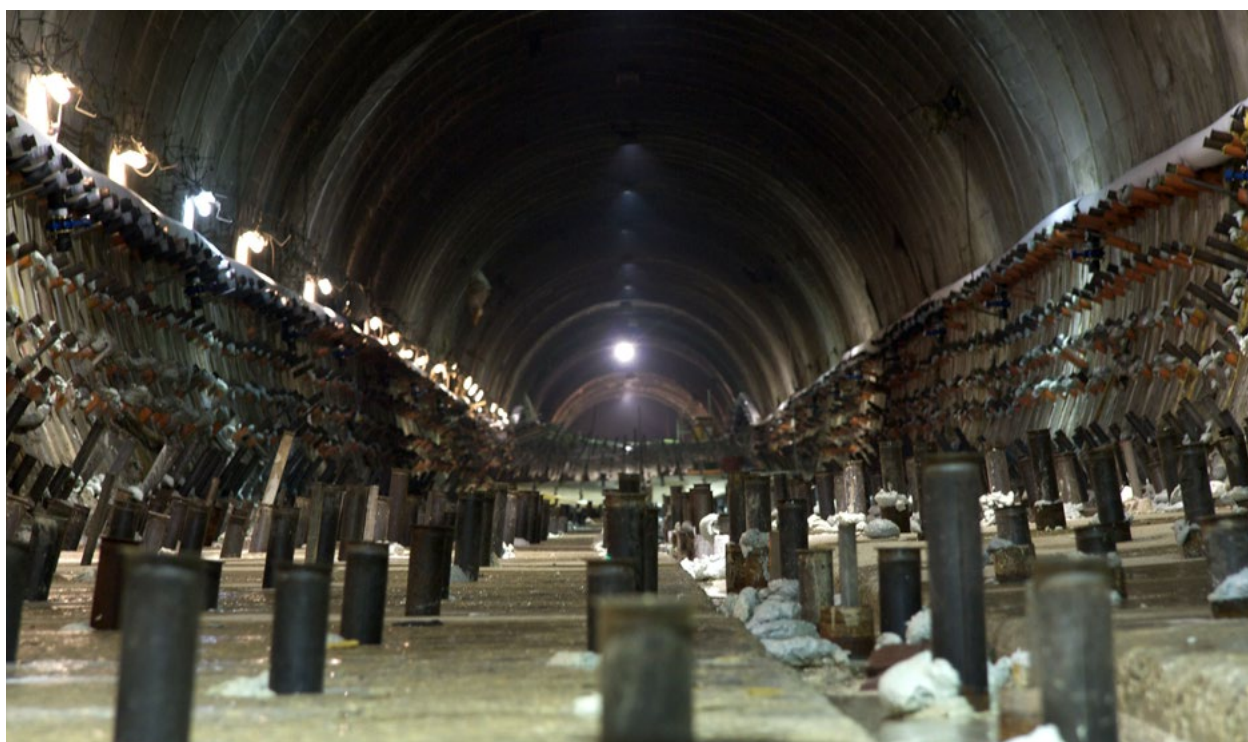
Fig. 11. Detail of the heads of the micropoles in the reverse arch.
