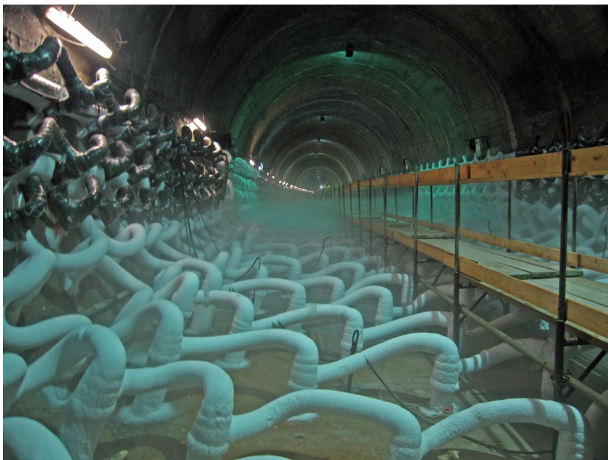
Fig. 1. Wide-angle view of the Cassia - Monte Mario (Rome) tunnel; freezing in the reverse arch and piers.
