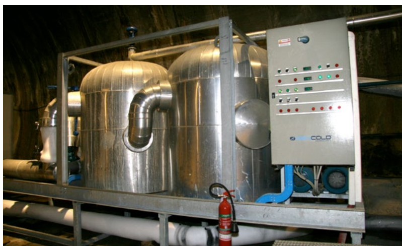
Fig. 6. Cold brine tanks and pump units.
