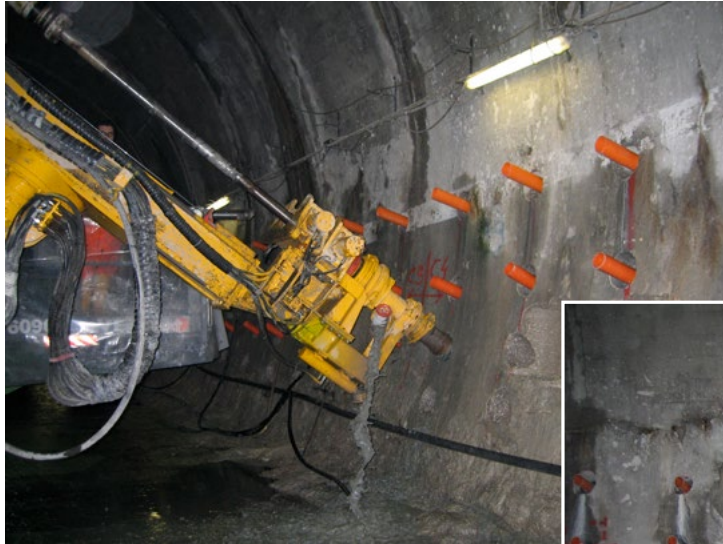
Fig. 3. Perforation in the piers for installation of the freezing (and thermometric) probes)
