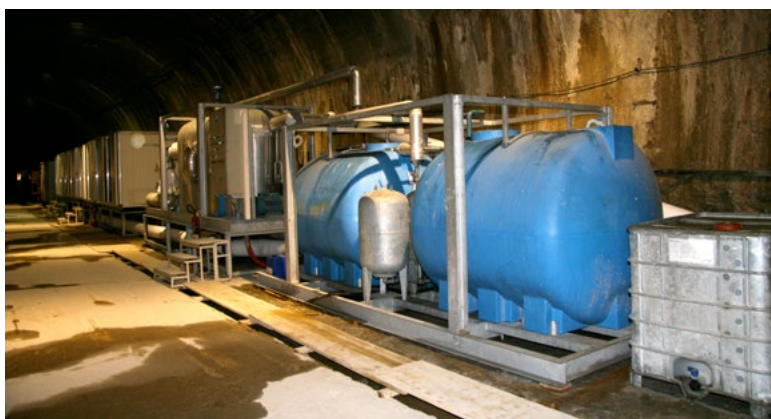
Fig. 5. Storage tanks for un-chilled brine.
