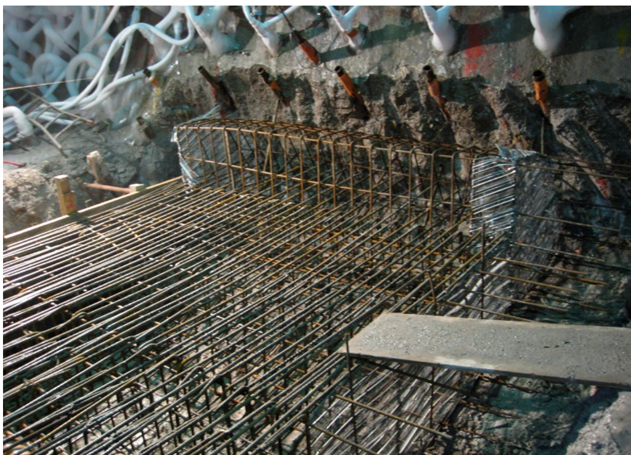
Fig. 18. Slab under reconstruction; assembly of reinforcement cage for final pouring.
