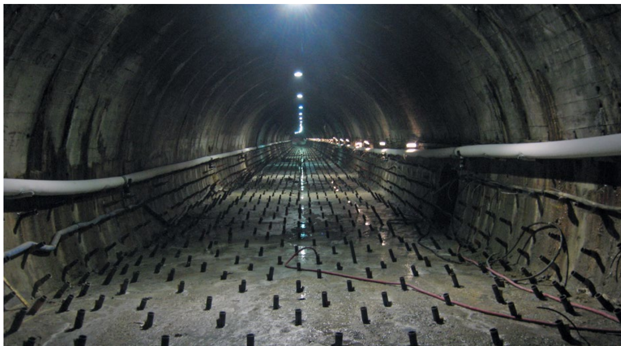
Fig. 10. Overview of the section of tunnel with micropoles ready to receive the probes.
