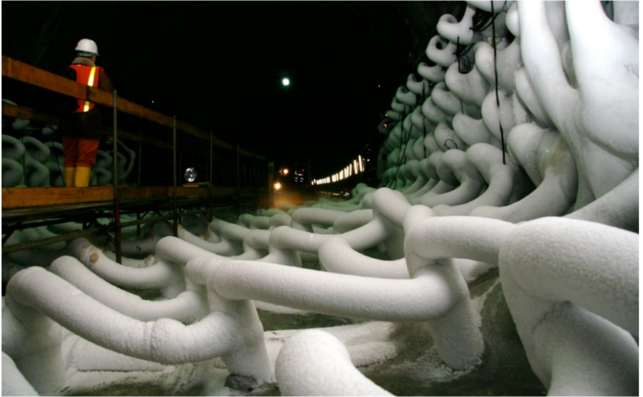
Fig. 16. Detail of the heads with the connecting sleeves; freezing field.
