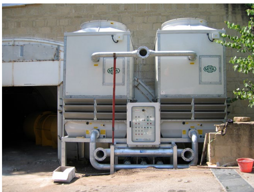
Fig. 9. Evaporation towers installed outside the tunnel.
