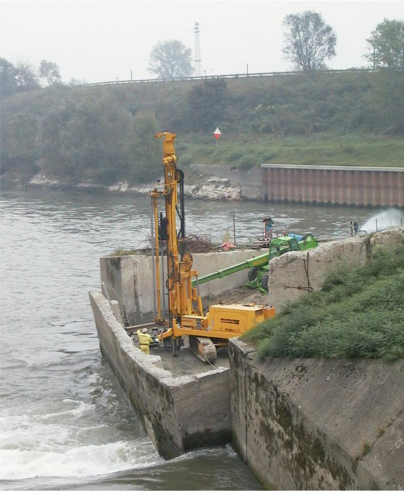
Fig. 4. Sonda P 1500 ESCR Jet Grouting.
