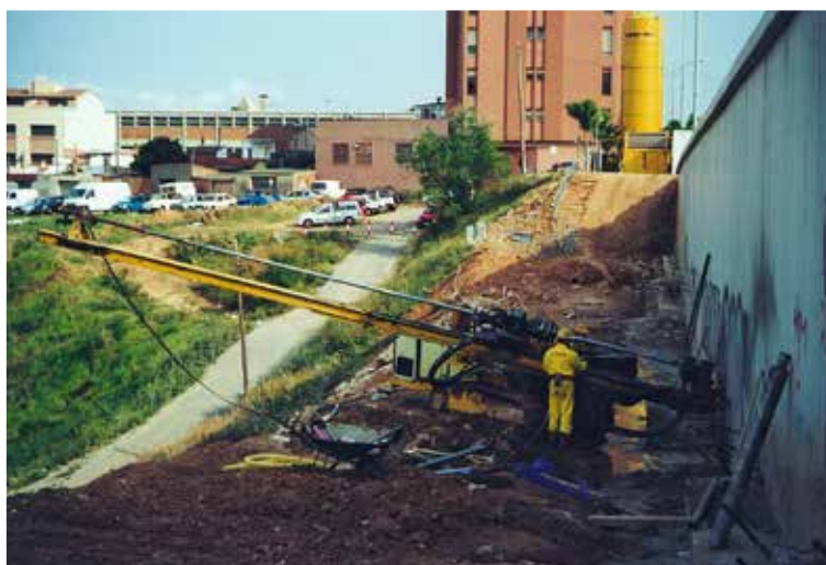
Fig. 10. PRP 105 drill rig during consolidation of the foundations
