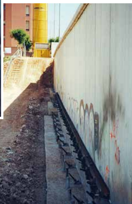
Fig. 9. Detail of load-sharing beams.
