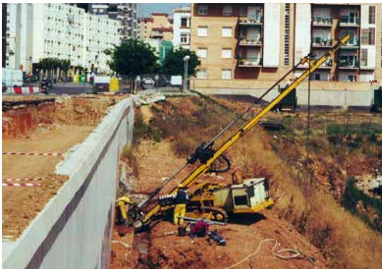
Fig. 6. PRP 105 drill rig during the anchoring of foundation beam.
