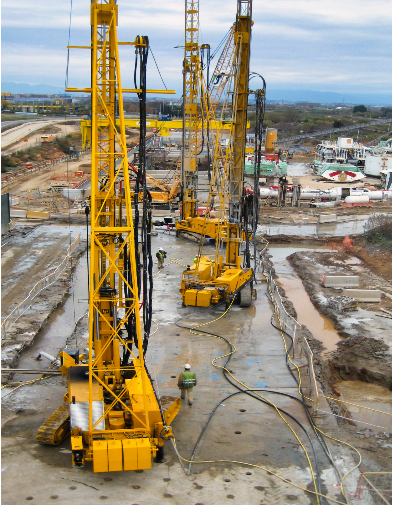
Fig. 10. PACCHIOSI P1800ECS2 drill rigs on work platform
