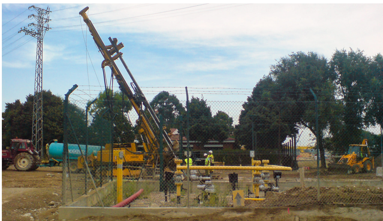
Fig. 7. PACCHIOSI P1500ES drill rig at work for sub-vertical treatments
