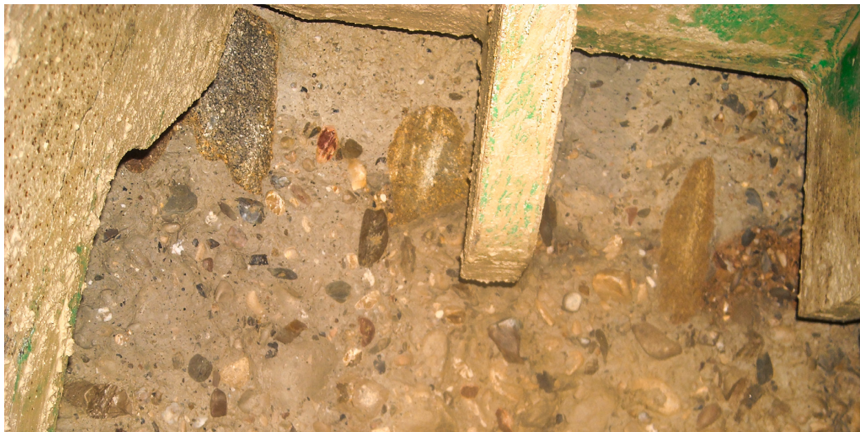
Fig. 6. View of good Jet Grouting soil treatment as present in front of TBM cutting head
