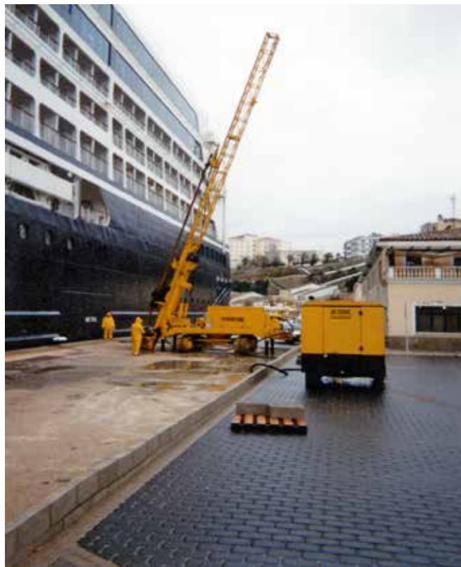
Fig. 3. P 1500 EC drill rig during Jet Grouting.
