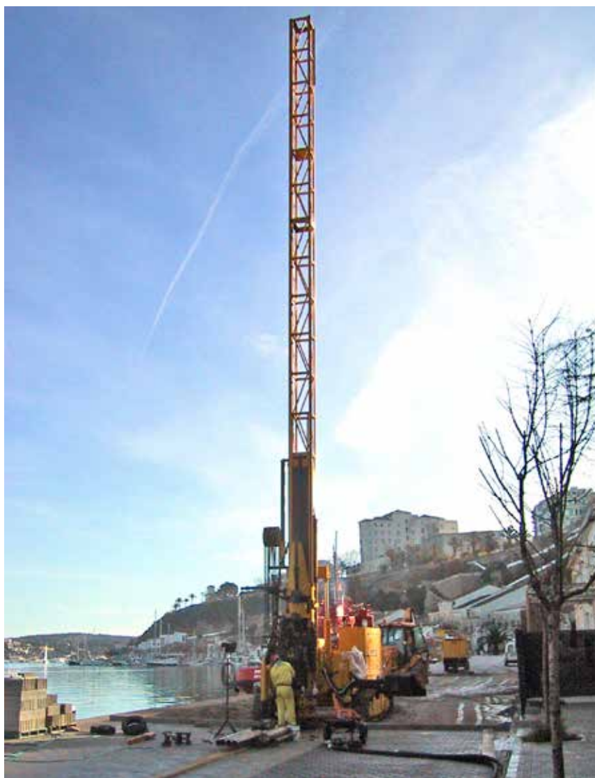
Fig. 1. P 1500 EC drill rig on the wharf.
