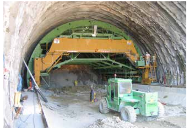
Fig. 15-16-17. Formworks for pouring of the vault; preparation in the open, carriage into the tunnel, works in progress.
