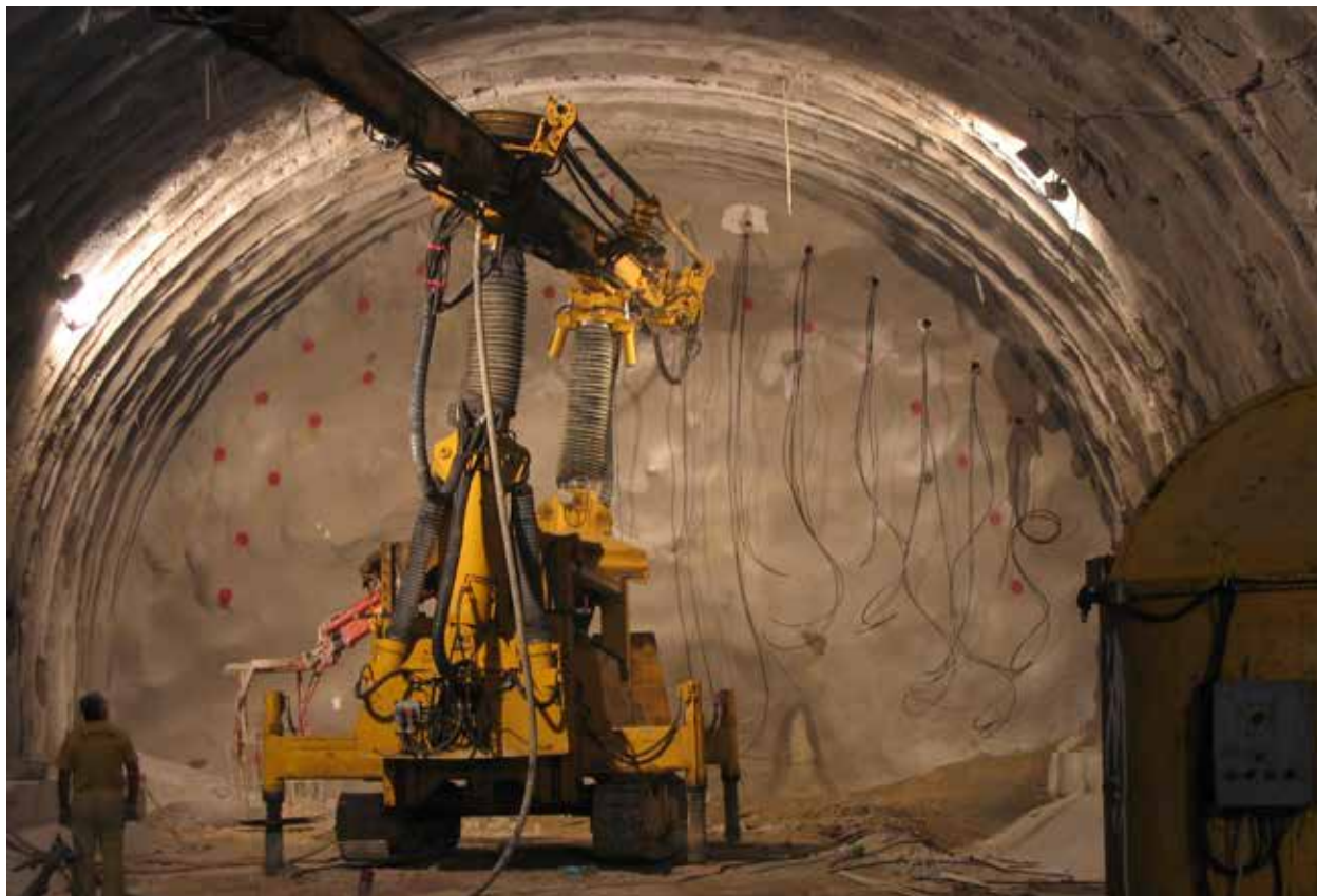
Fig. 12. Nailing of the front with PACCHIOSI P1500TAF.
