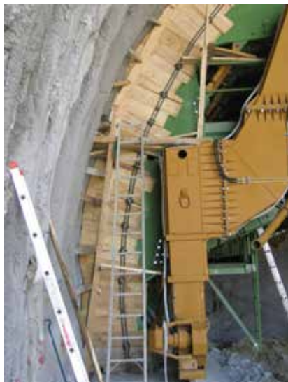
Fig. 18. "Damper" at the end built at the site for perfect adaptation to the profile of the preliminary covering already applied
