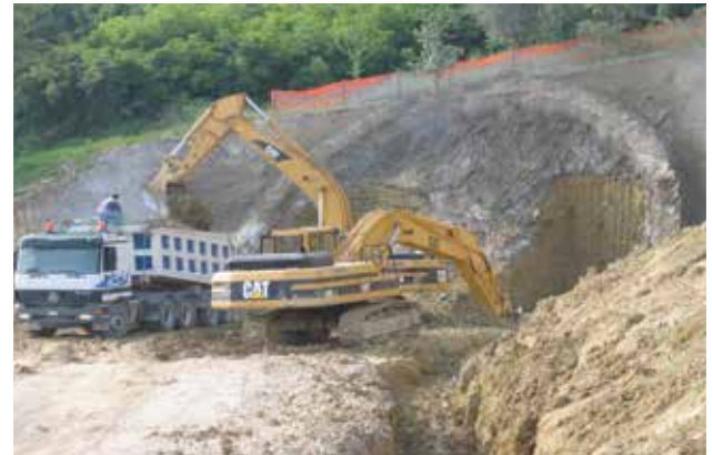
Fig. 10. Approach of excavation face at North entrance.
