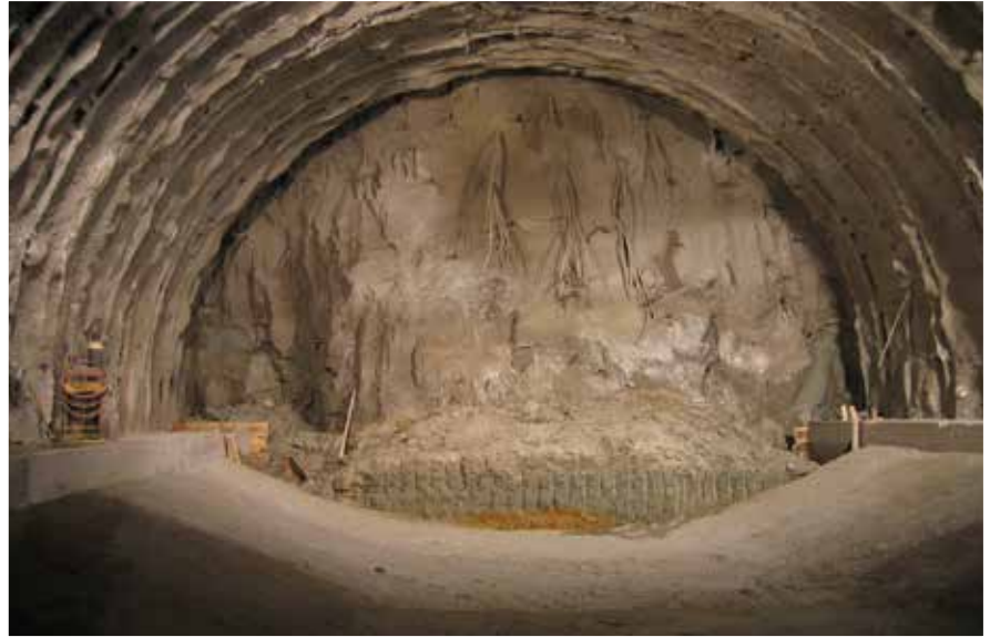
Fig. 14. Preliminary covering with reverse arch immediately after the front.
