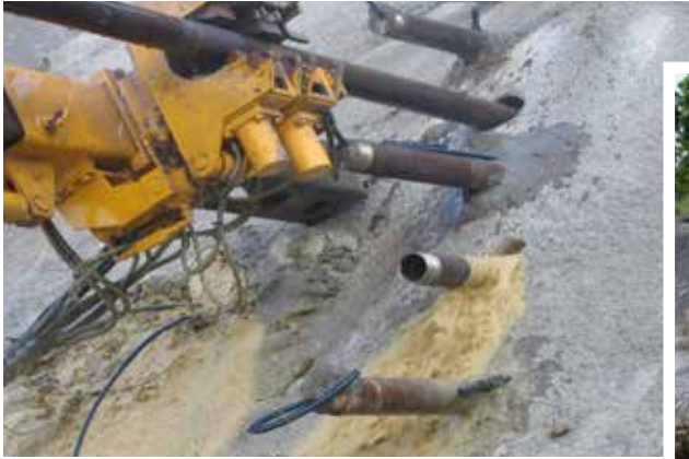
Fig. 8-9. Detail of construction and view of subhorizontal steel insertions preliminary to first attachment on the front.
