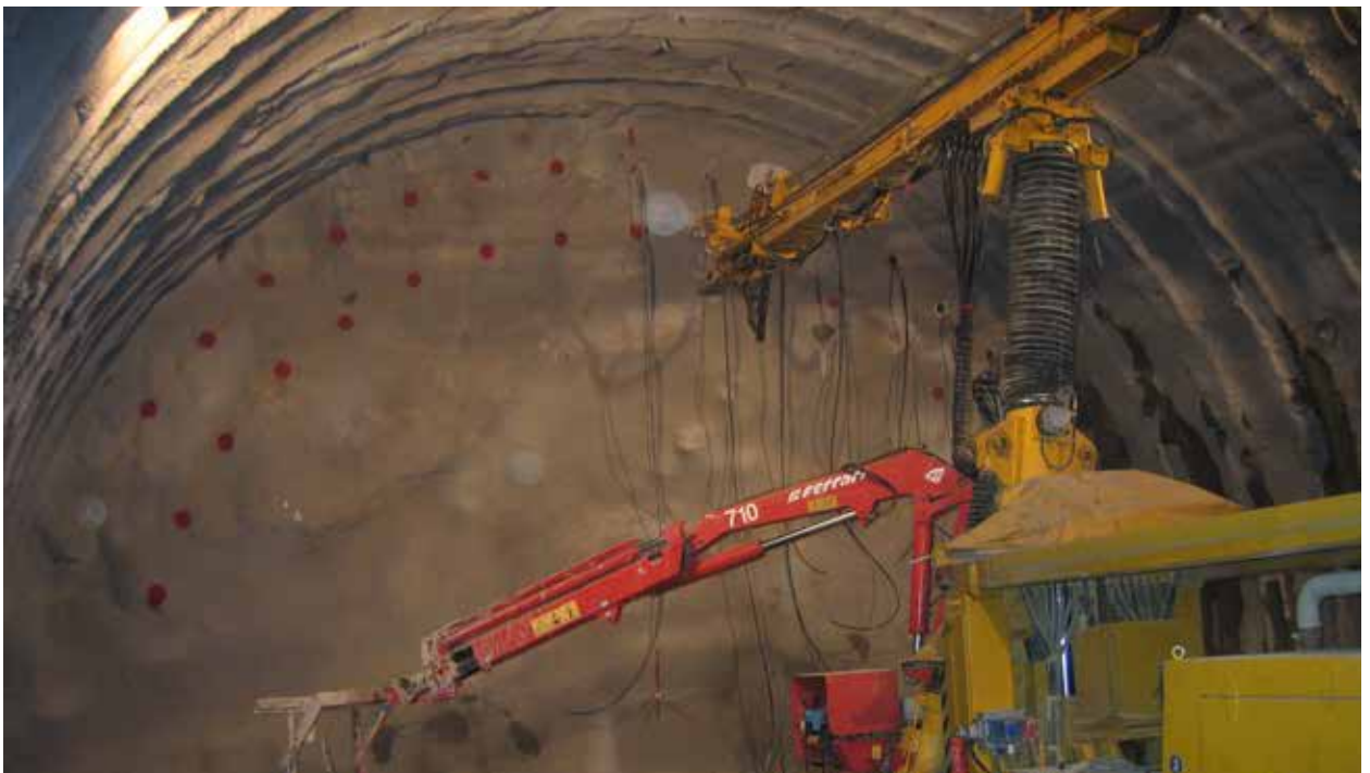
Fig. 11. PACCHIOSI P1500TAF drill rig executing the nailing of excavation face
