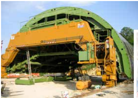
Fig. 15-16-17. Formworks for pouring of the vault; preparation in the open, carriage into the tunnel, works in progress.
