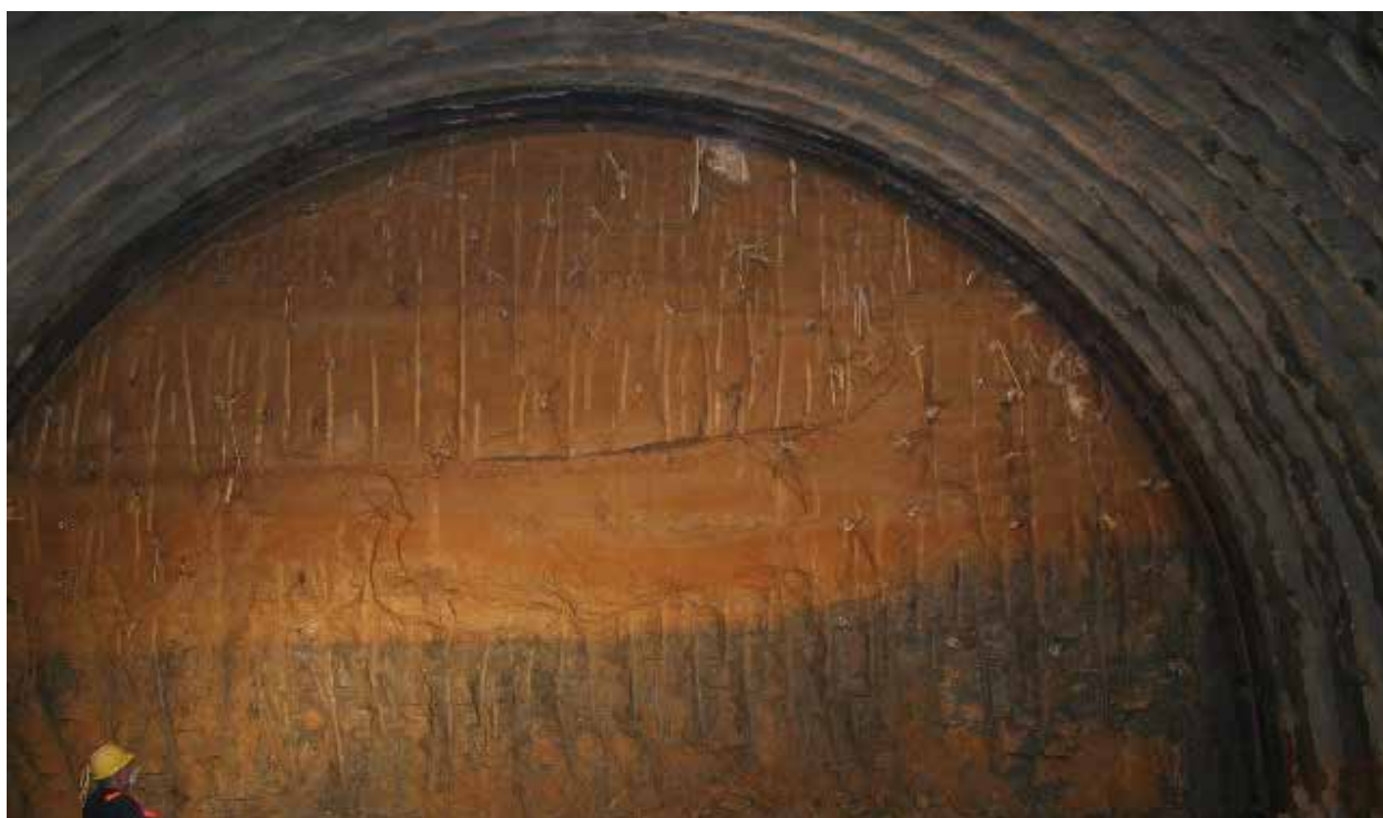
Fig. 13. Front of the excavation; the soil stratigraphy is visible.
