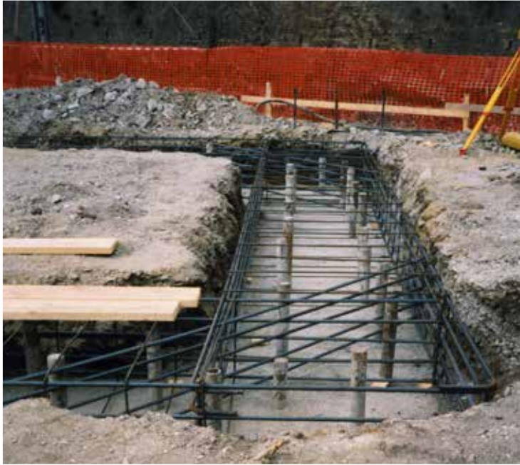
Fig. 4. View of the reinforcement of the columns composing the perimetral diaphragm of the well and perimetral beam.
