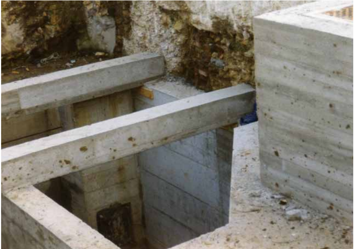
Fig. 9. Protection of shaft after completion.
