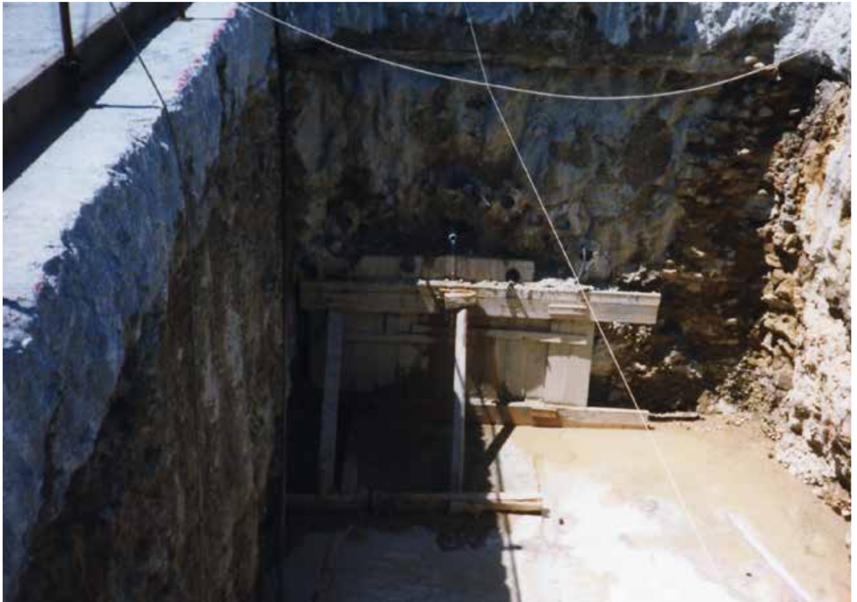
Fig. 5. View of the intersecting Jet Grouting columns and crowning beam.
