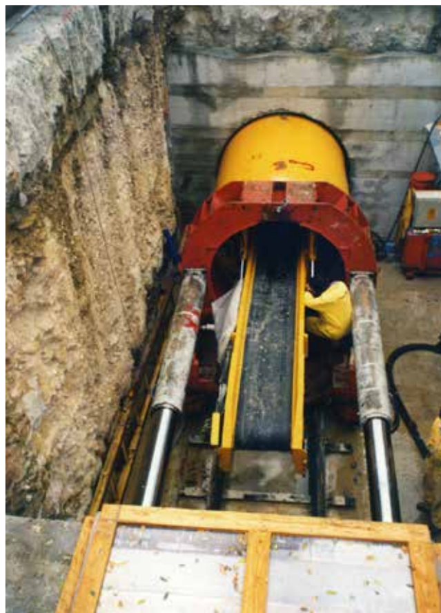
Fig.10. Insertion of an element of the minitunnel.
