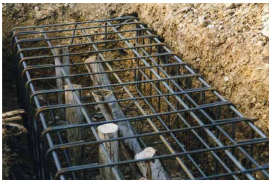
Fig. 15. Detail of the reinforced beam at the top of the A-frame.
