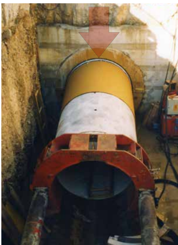
Fig. 12. Pipe pusher with intermediate station. The arrow shows the element preceding the intermediate pushing station (in yellow).
