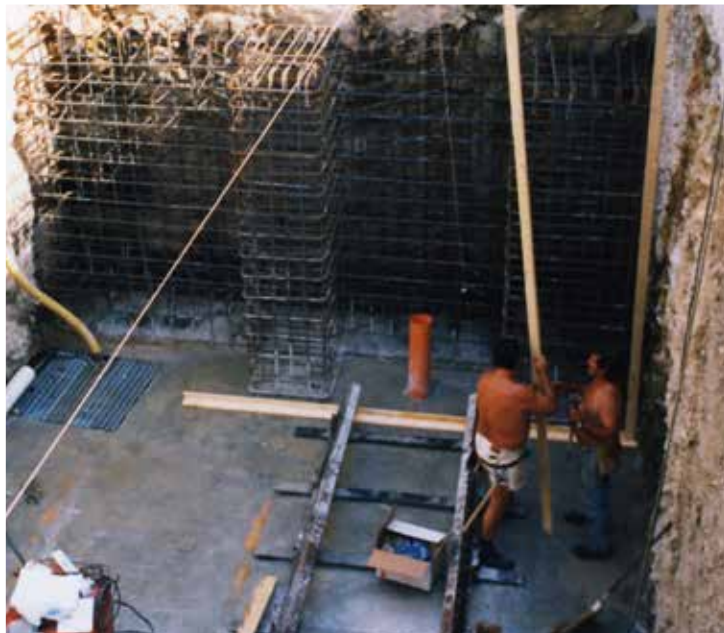
Fig. 6. View of the bottom cap on the track on which the tunnel elements will move.
