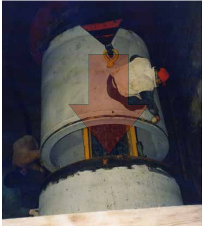
Fig. 13. Picture of two section of the tunnel on which a wooden bearing was applied (shown by the arrow).
