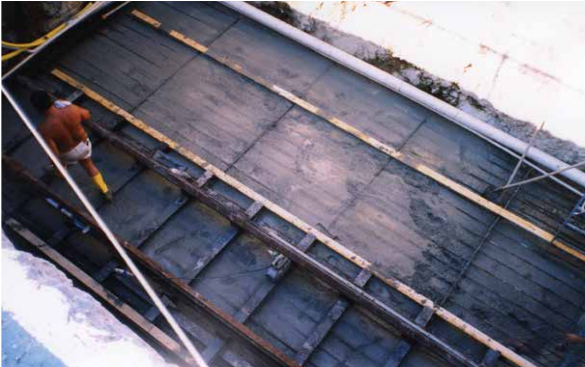
Fig. 6. View of the bottom cap on the track on which the tunnel elements will move.
