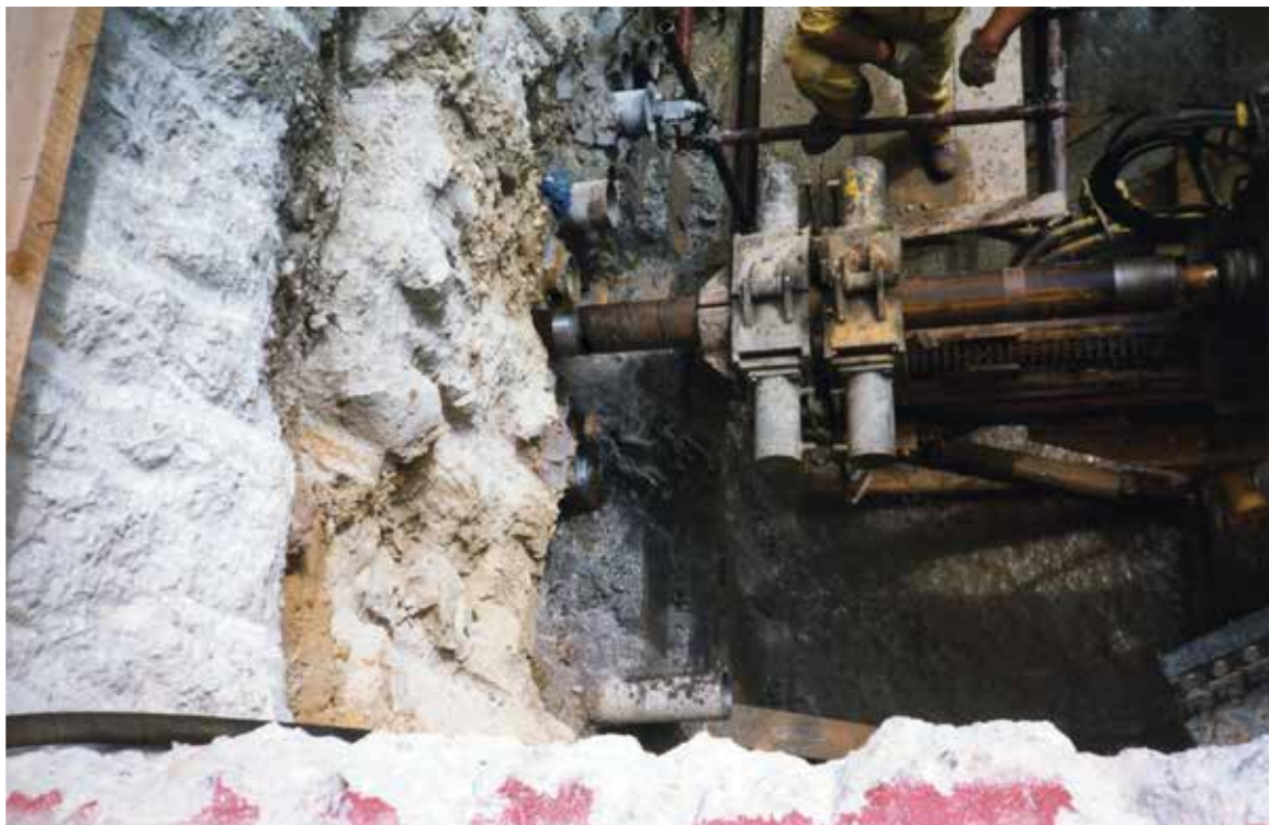
Fig. 2. Insertion of the supporting piles in the roof of the minitunnel.
