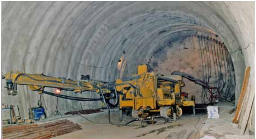
Fig. 7. Works on the entrance, lay-out of the nails and micro-piles.
