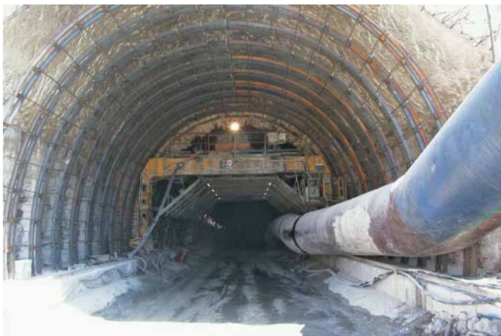
Fig. 5. Stage of application of final lining.
