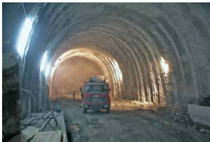
Fig. 4. View of the tunnel with preliminary lining.
