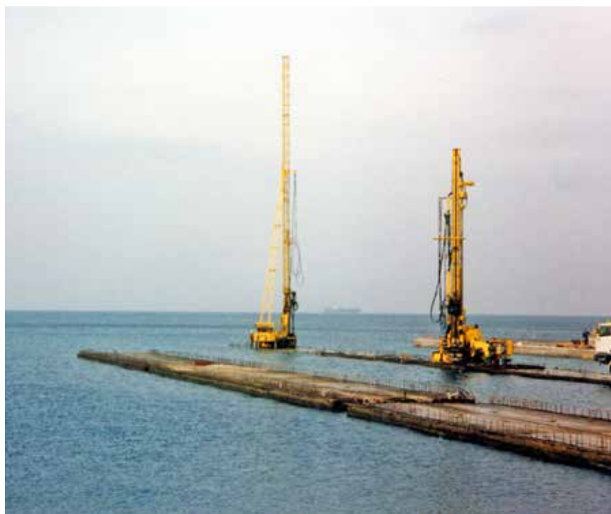
Fig. 7. P 1500 EC and PRP 1500 ECSdrill rigs during the execution of works.
