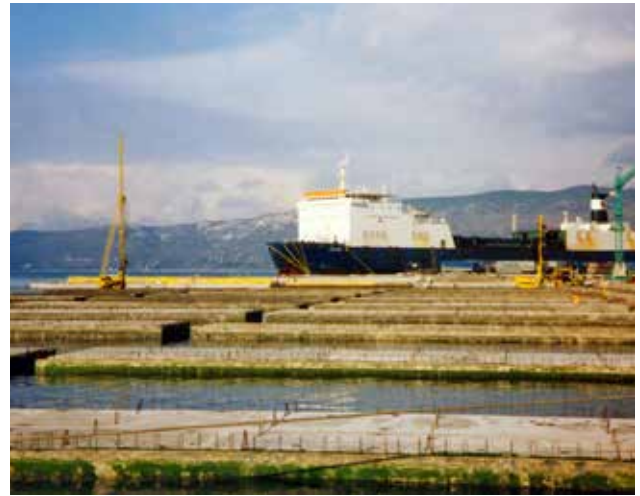
Fig. 8 - 9. View of cellular caissons(above) and preliminary holes (left).
