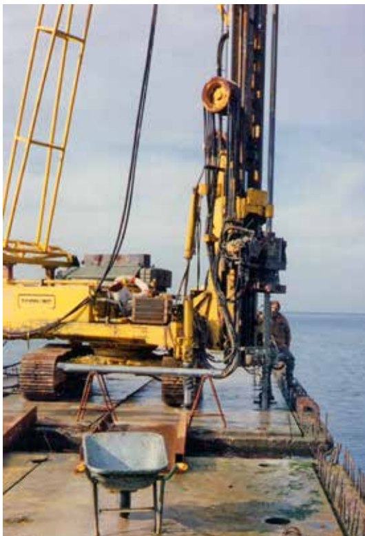
Fig. 10. P 1500 ES drill rig performing Jet Grouting.
