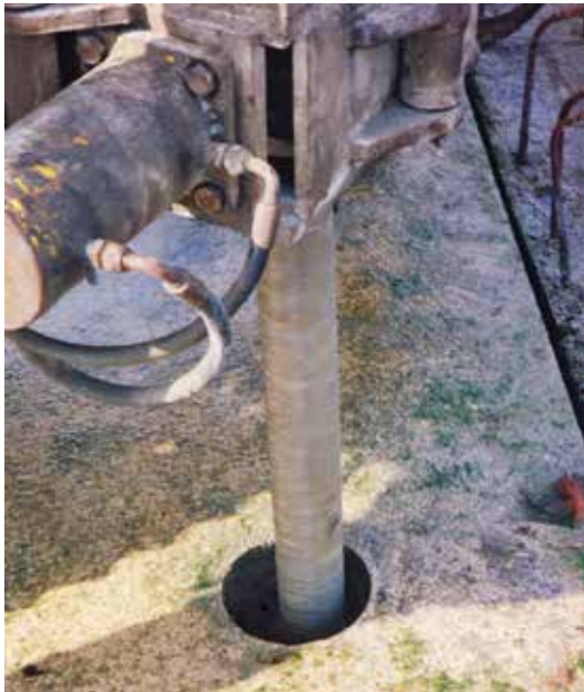
Fig. 8 - 9. View of cellular caissons(above) and preliminary holes (left).
