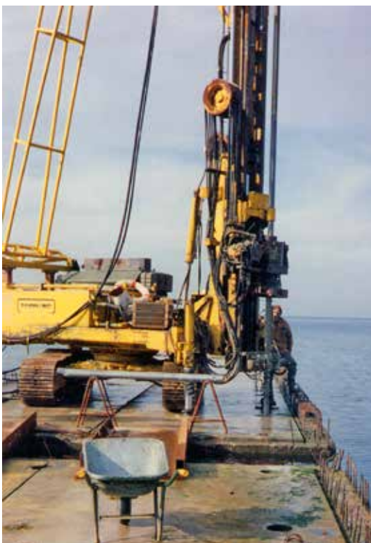
Fig. 10. Sonda P 1500 ES Jet Grouting.
