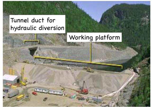
Fig. 6. View of the worksite.
