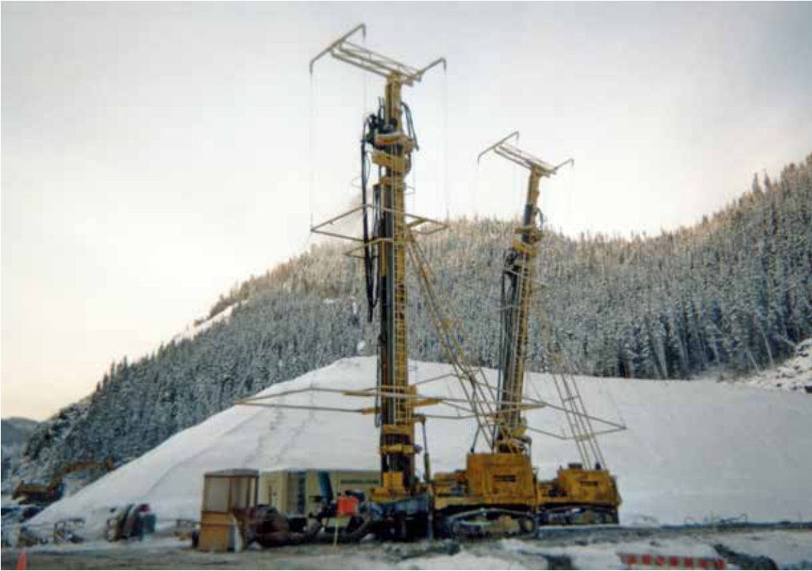
Fig. 8. P 1500 drill rig with rod-charger.
