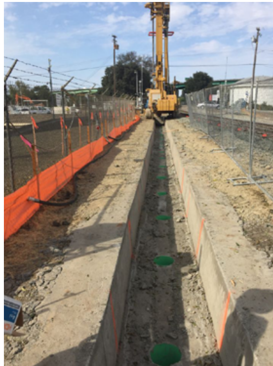
Fig. 18, - P 1500 drilling machine in action
