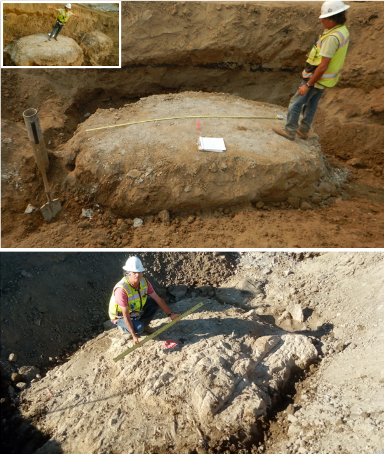
Fig. 11 | 12. Columns with variable geometry made in the test field.
