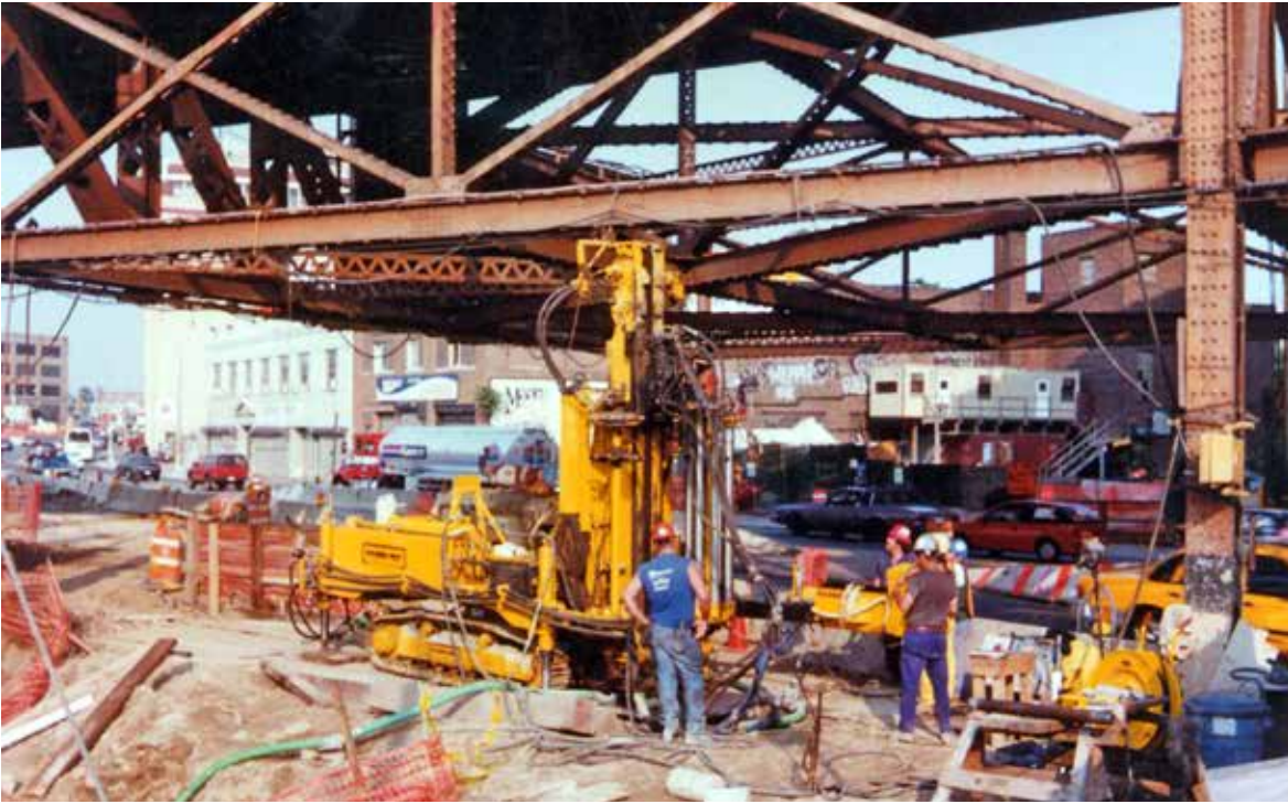
Fig. 4. P 1000 probe with short mast and automatic loader.
