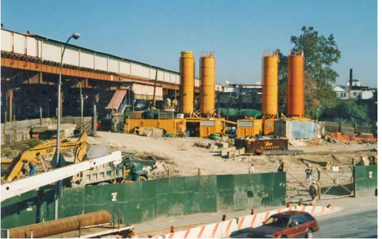
Fig. 12. View of the worksite.
