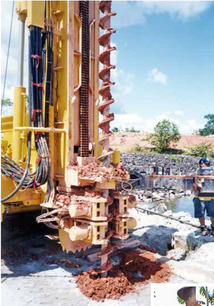
Fig. 11. Perforation using propeller rods to lay piping in pvc.
