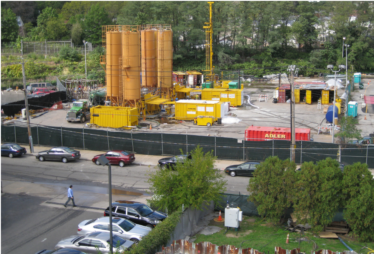
Fig. 10. PACCHIOSI Jet Grouting plant installations.
