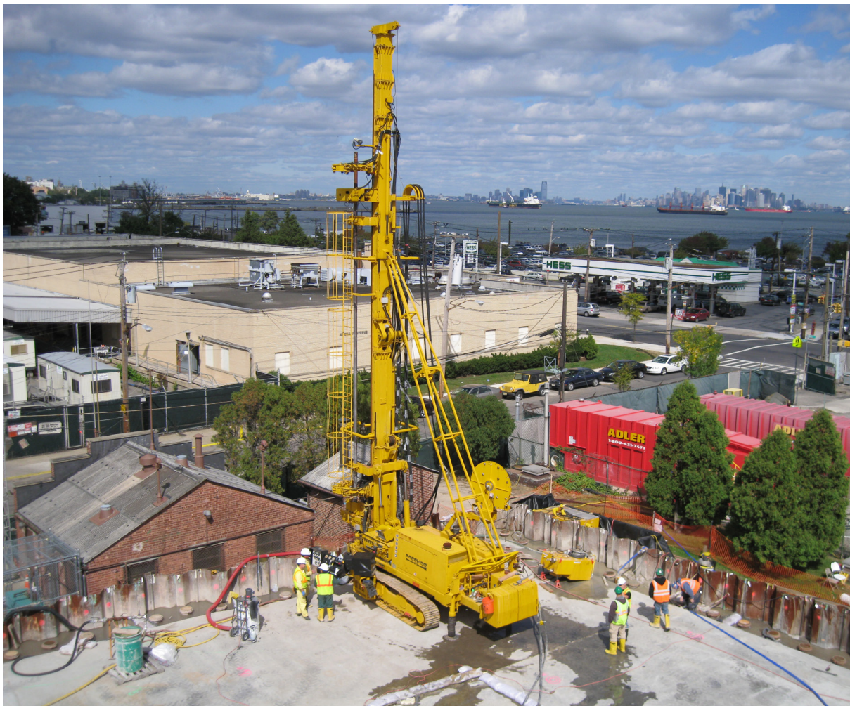
Fig. 1. Former Clifton OU-1 MGP site.
