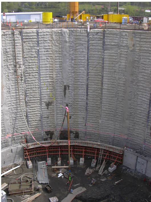
Fig. 9. View of circular excavation of the Pump Station shaft..
